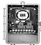
Grasslin timer installed on Snowmass Mountain heaters.
