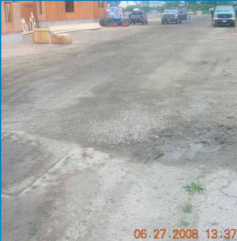
Before (during inspection)
