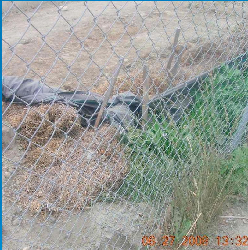
Before (during inspection)
