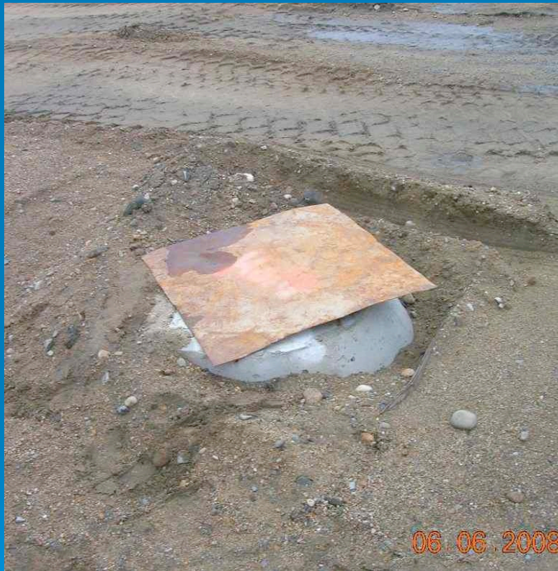
Before (during inspection)
