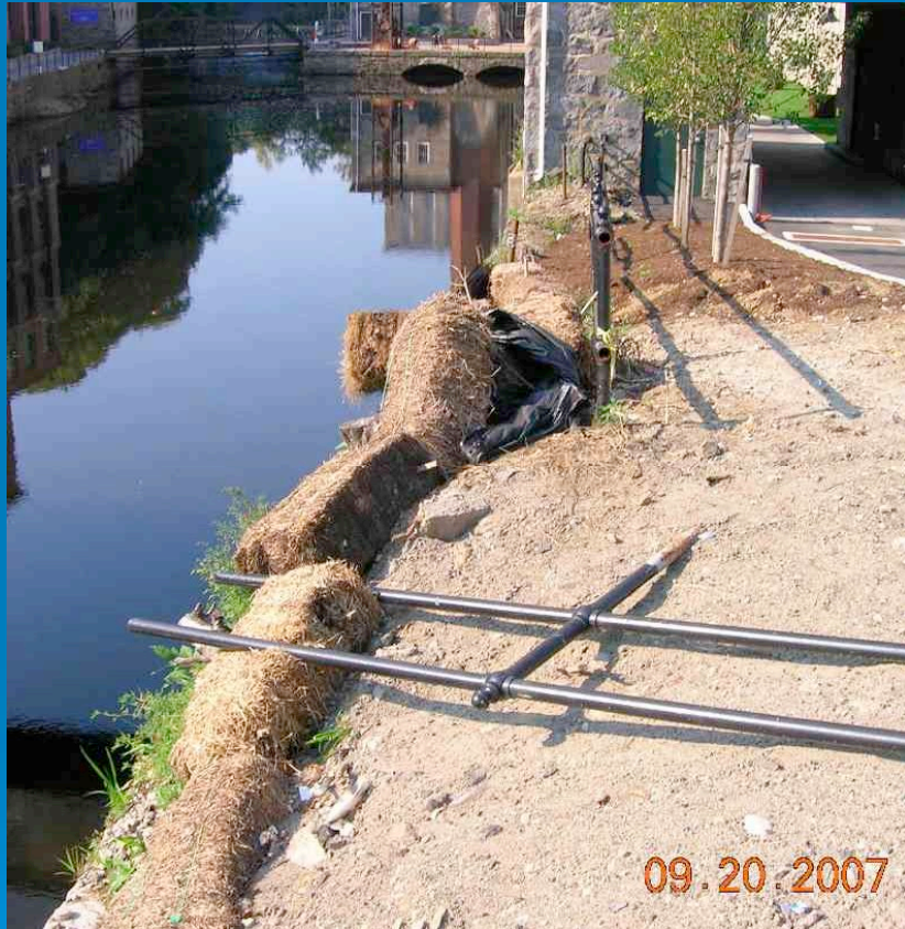
Before (during inspection)
