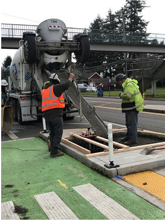
Traffic signal pole footing
