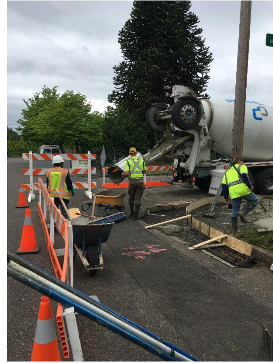
Pavement and ADA ramps
